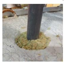
should be used to pack around the pipe. This should be installed within the QuelCast, above the rubber smoke seal up to the top of the concrete floor slab.
