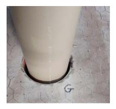
Where a smaller diameter pipe is used such as a 75mm diameter in a QuelCast110 and always in the case of a QuelCast50 and cable bunches, a 45kg/m3 rockfibre insulation
