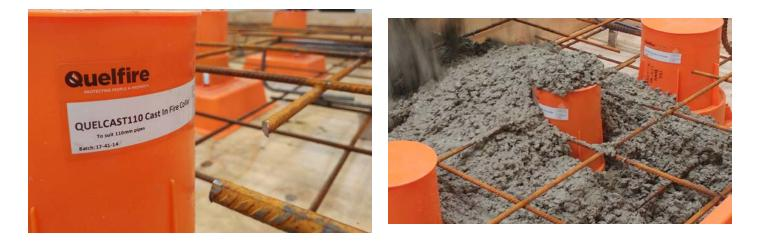
Once cured, remove the shuttering formwork - note that the corners of the QuelCast may break off depending on the 10. fixings used - this does not affect the performance of the product and is in fact to facilitate easy removal of the shuttering formwork.
