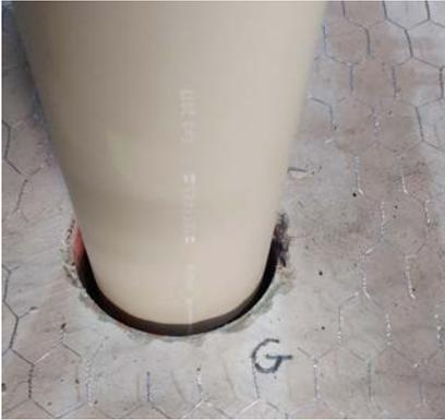
Where a smaller diameter pipe is used such as a 75mm diameter in a QuelCast110 and always in the case of a QuelCast50 and cable bunches, a 45kg/m<sup>3</sup> rockfibre insulation
