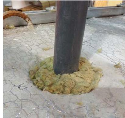
should be used to pack around the pipe. This should be installed within the QuelCast, above the rubber smoke seal up to the top of the concrete floor slab.
