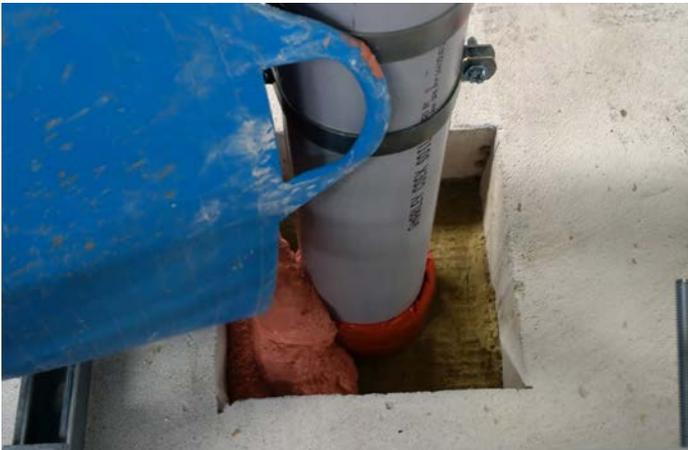
QWW CE Marked Intuwrap installed in an oversized hole sealed with QF2 Fire Protection Compound in concrete slab
