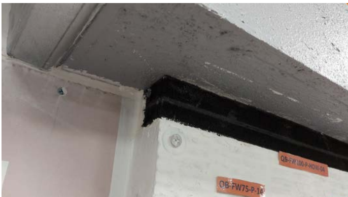
QI Intufoam used in conjunction with QuelStop Fire Batt to allow for deflection in a head of wall seal
