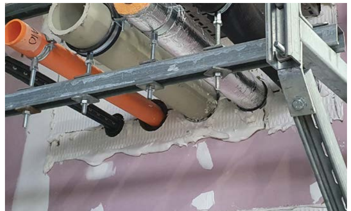
Example Single Side Access Batt Installation as viewed from the non-accessible side showing liberal amounts of sealant.
