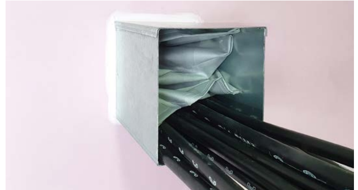
QFP QuelStop Intumescent Fire Pillows Installed in Steel Cable Trunking
