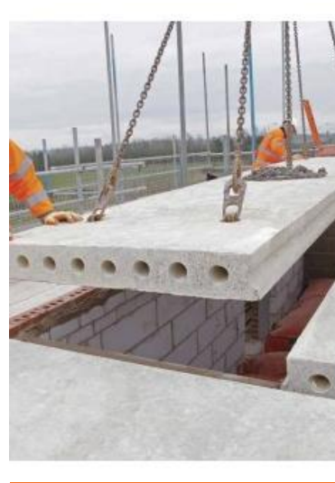
Hollow Core Slab (Pre-Cast Concrete Slab)
