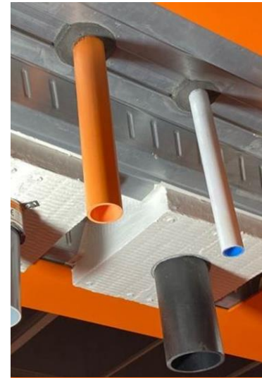
Steel Profiled Deck (Composite Deck)
